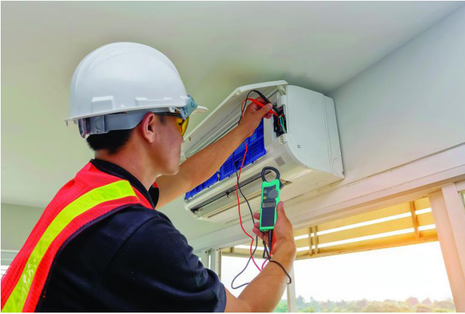
A worker installs a unit that provides air conditioning and heat.
