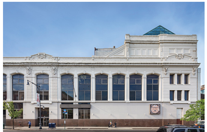
Billie Holiday Theater infrastructure improvements included adding new boilers and air-conditioning units that work with the building's existing geothermal system. Photo: Francis Dzikowski/OTTO
