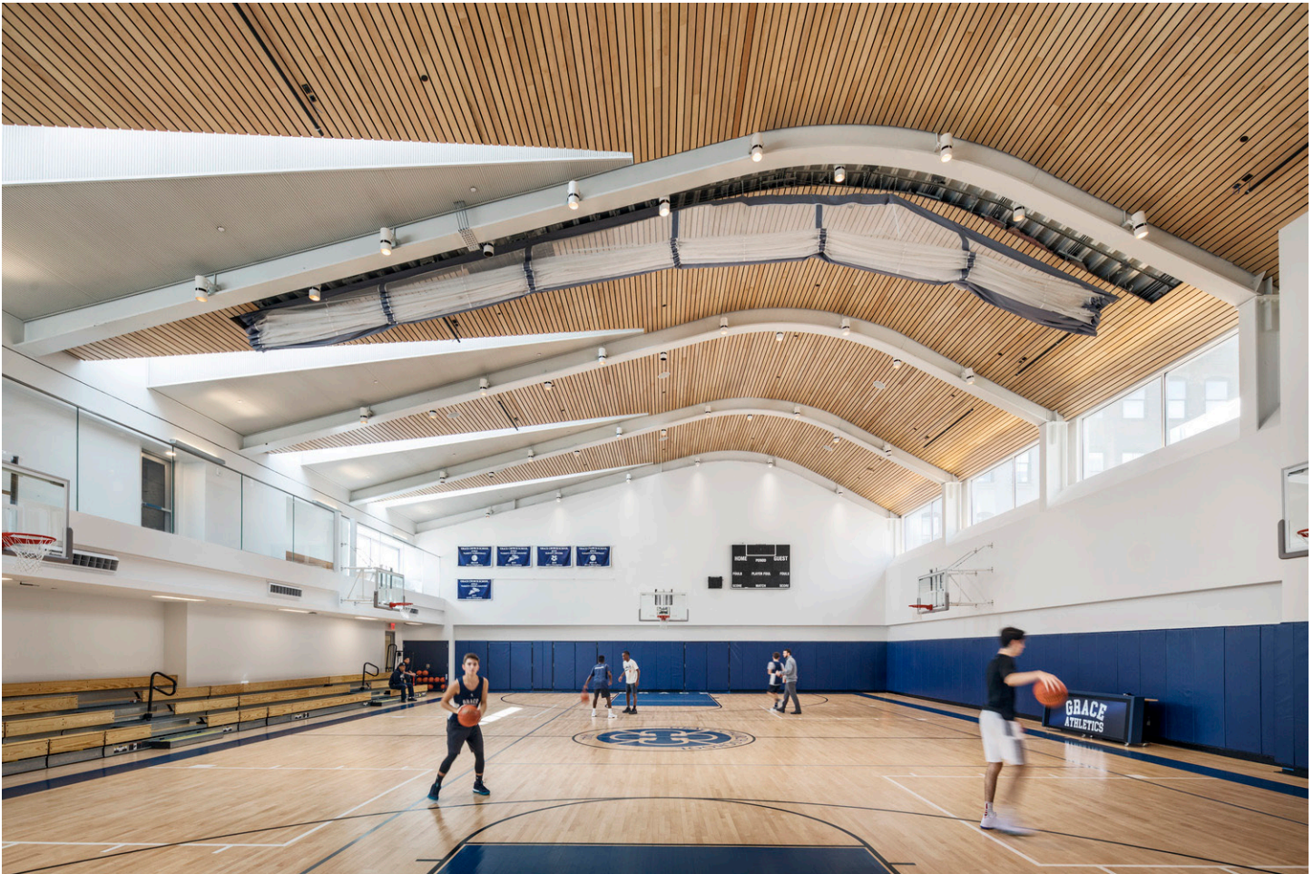
A new gym, designed by Murphy Burnham & Buttrick for the Grace Church School in Manhattan has a boomerang-shaped roof invisible from the street. Courtesy Francis Dzikowski/Otto
