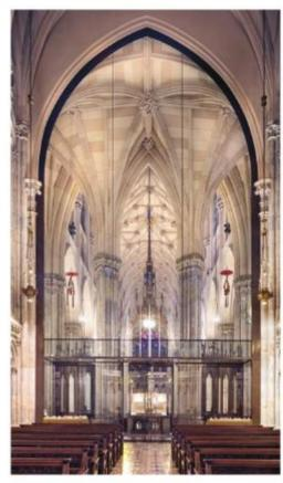
Glass sliders enable St. Patrick's bronze entry doors to open (top left and right) without wasting energy. A floor-to-vaulted ceiling glass wall (above) acoustically seals off the Lady Chapel.
