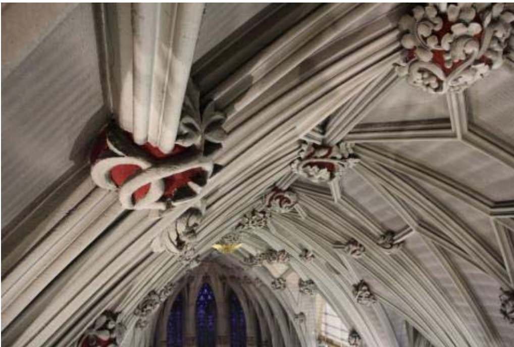
Each of the red decorative bosses that adorn the ceiling have a unique design. The plastered ceiling vaults will soon be scrubbed clean and repainted.
