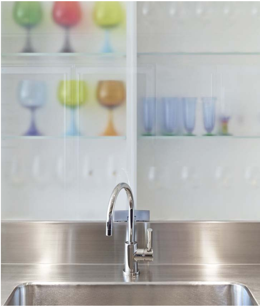
Above: The glassware cabinet over the sink is clad in 5/16th inch sandblasted tempered glass. The clients' glassware collection creates a colorful backdrop.
