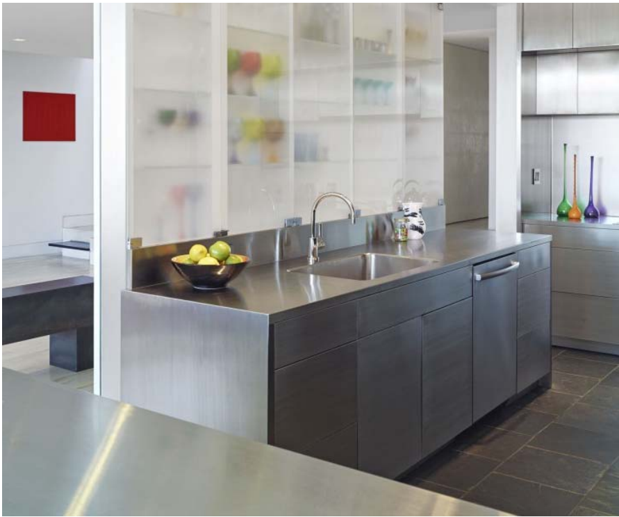
Above: The stainless steel sink was welded to the counter and backsplash. The weld was then ground smooth and brushed integrating the sink into the unit. The architects used 16-gauge stainless steel sheets with a #4 brush finish. The grain runs vertically to match the refrigerator and wine cooler. While pleasing to the eye, brushed stainless steel with welded corners requires regular maintenance; the owners regularly apply an aerosol stainless-steel cleaner with a cotton cloth to keep the design clean and polished. "To address this issue, there is a chemical treatment that minimizes fingerprints, but it will change the hue of the stainless steel," Murphy says. "Alternatively, in the future, we would use a coarser brush finish."
