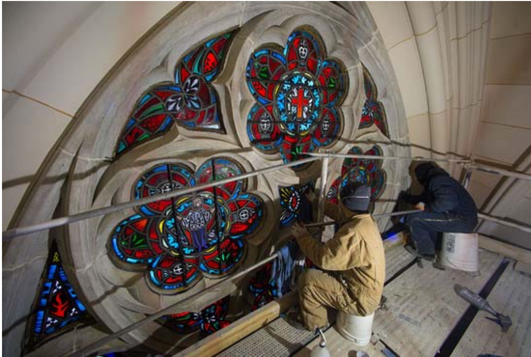
Angel Arias, left, and Hector Avila with the Botti Studio work to restore the stained glass windows near the ceiling of Saint Patrick's Cathedral.
